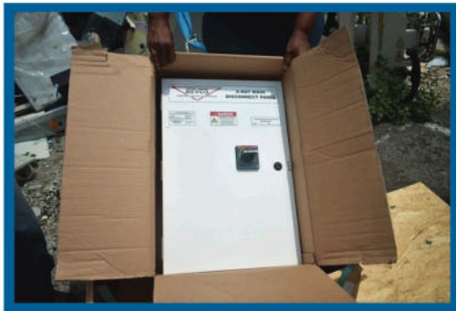
Photo showing a box with the X-Ray Main Disconnect Panel, which provides emergency shut down, undervoltage protection and overcurrent protection for the machine.
