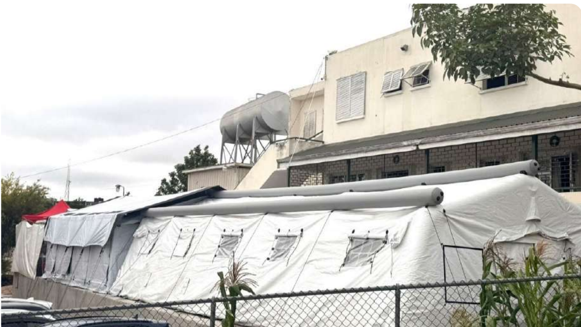
A section of the field hospital at the Mandeville Regional Hospital
