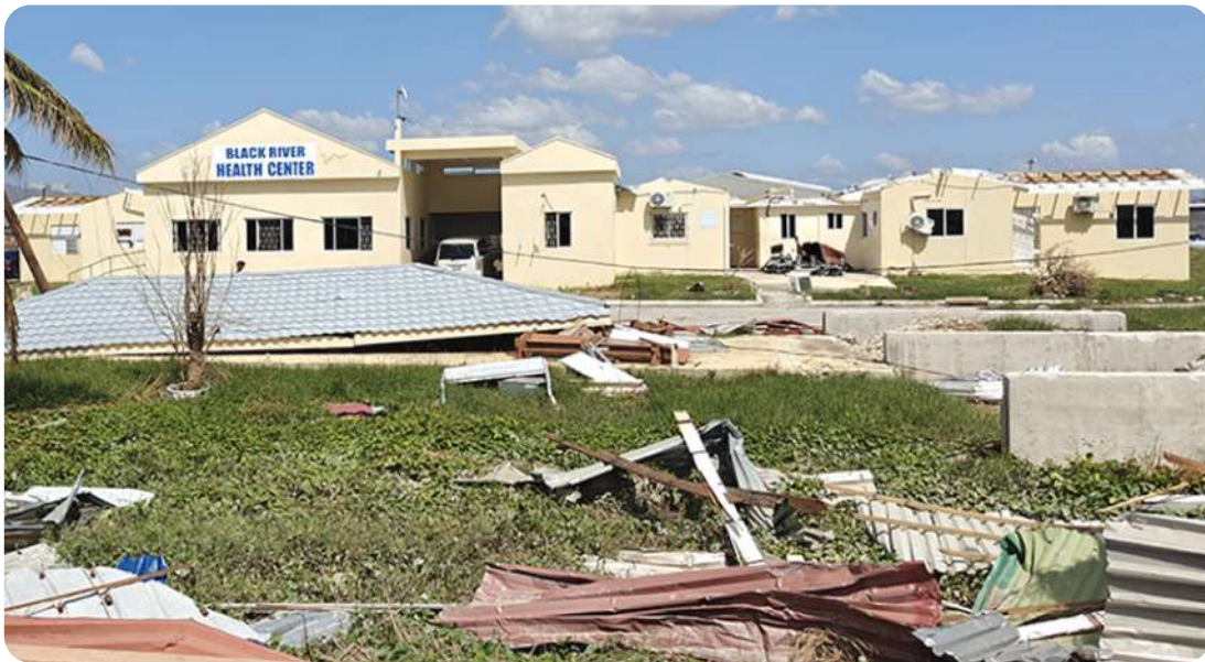
Hurricane Melissa Emergency Relief Effort – Black River Health Centre (Before)
