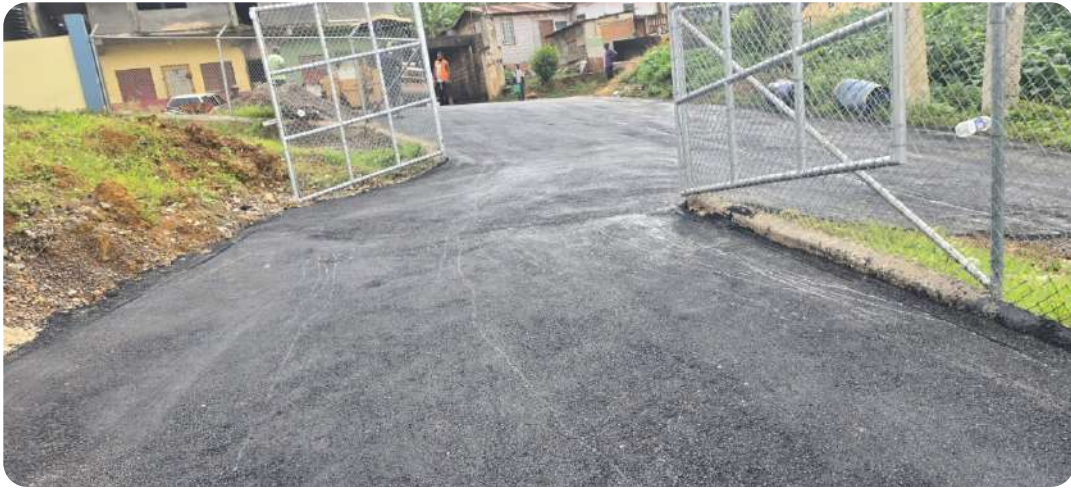
Craighead Health Centre - Parking and Boundary Fencing, Operation Refresh
