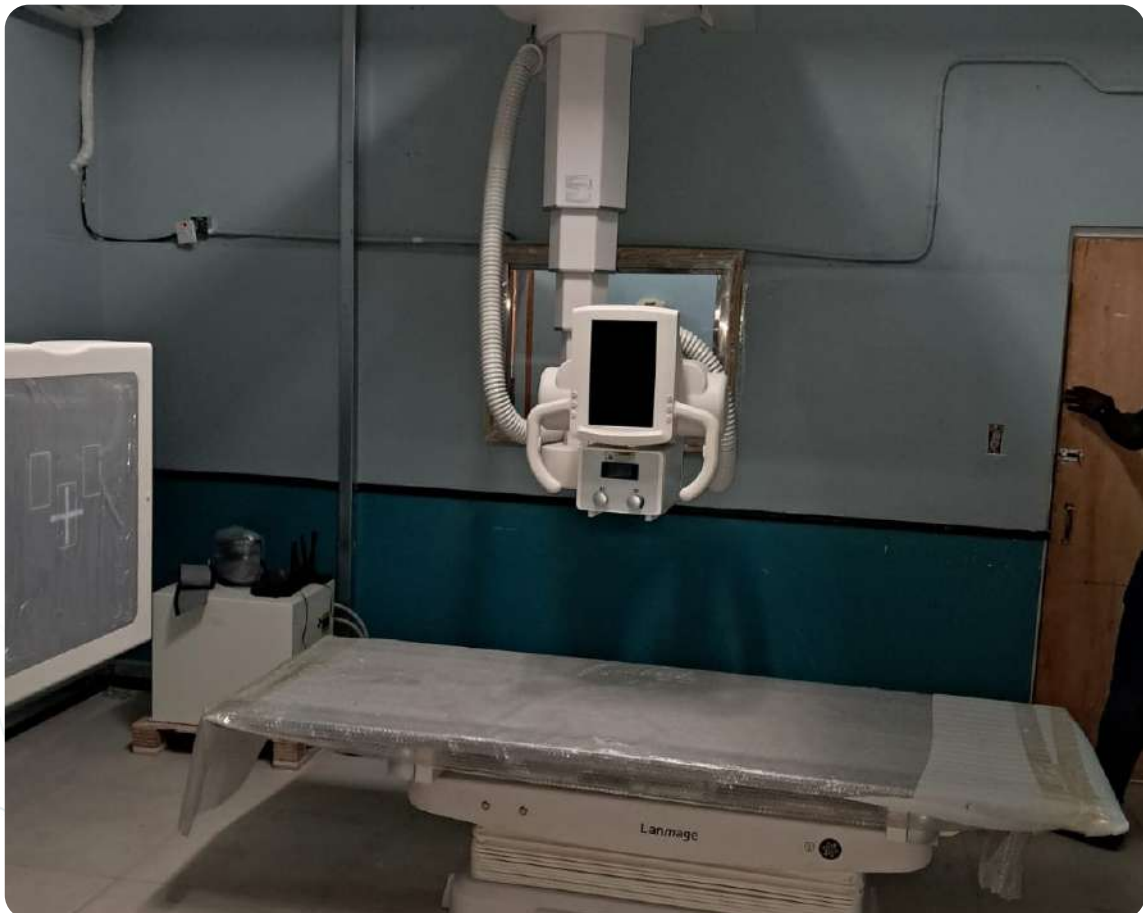
Installation of new X-Ray machine
