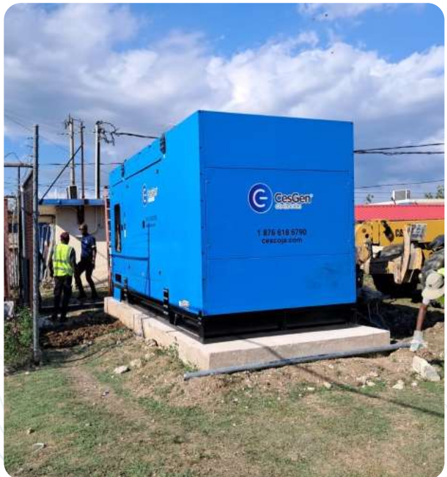
Installation of 750 KVA generator
