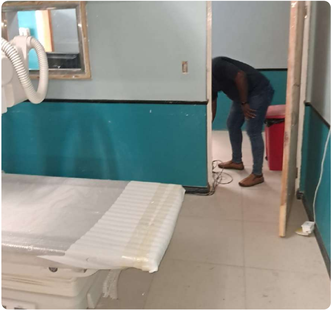
Renovation of X-Ray suite
