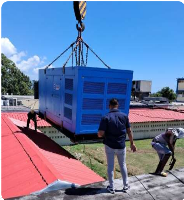
Installation of 750 KVA generator
