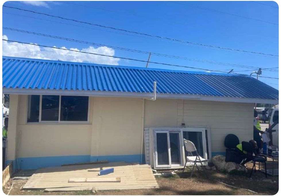
Installation of a base to facilitate use of a compactor to dispose of domestic waste
