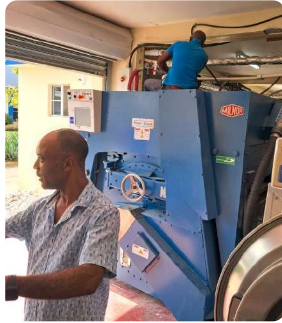
Installation of new washing machine at the laundry
